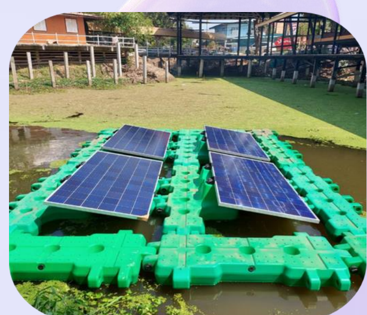
(1) Floating device, 3 kW PV Module, and DC Cable Power
