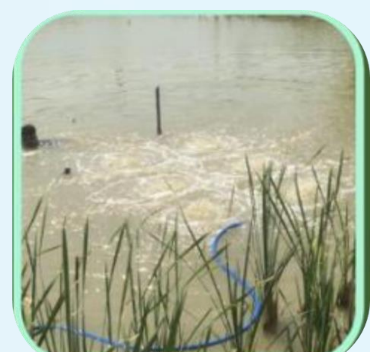
(10) Water Treatment Pound
