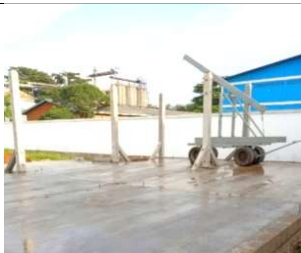
Hand crane raising posts on the ground slab.
