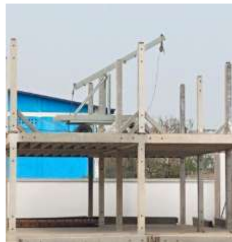
Hand crane lifting posts and beams from the ground and posing them at the 2 nd floor
